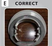
**E & F**: Ensure sealant ring provides coverage at front of opening as shown in Photo E & F.
