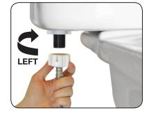
B: REMOVE OLD LOCKNUT Below tank, twist locknut to the left (clockwise) to remove from fill valve.
